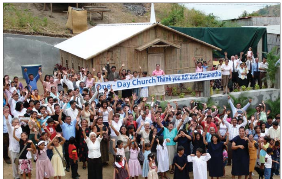
The first One-Day Church was completed in June, outside of Guayaquil, Ecuador. The building was assembled in a single day and ready for a service that night.
